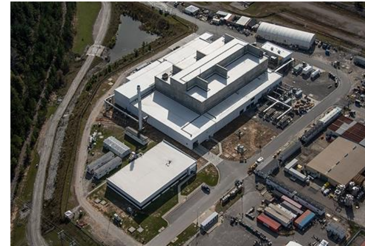
Salt Waste Processing Facility
