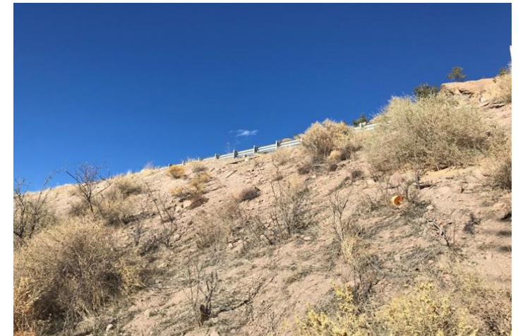
Cliff Alongside Transportation Route in Los Alamos
