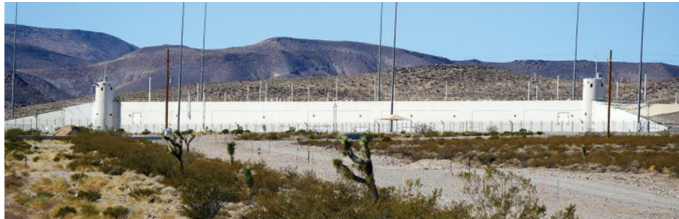
Device Assembly Facility
